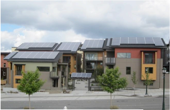
zHome at completion
