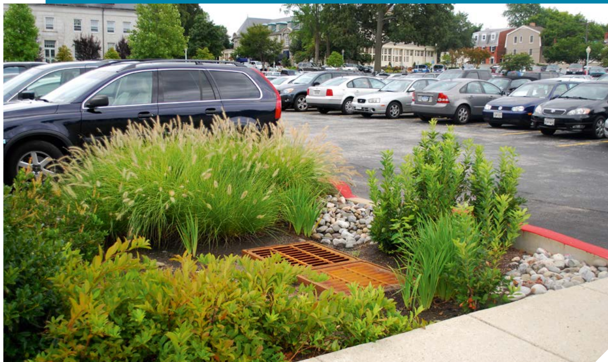
Rain garden in a parking lot.
