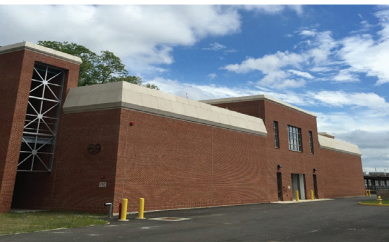
The AlexRenew Centrate Pre-Treatment Facility
