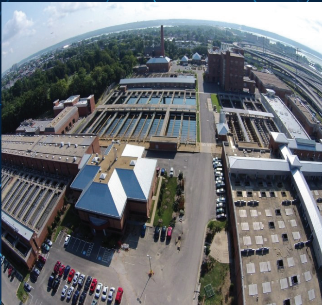
Located in Alexandria, Virginia, Alexandria Renew Enterprises is one of the most advanced water resource recovery public utilities in the United States.
