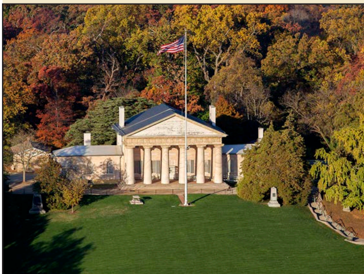
Arlington House, The Robert E. Lee Memorial. NPS Photo.
