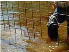
"Prongs" on the bottom of the fencing to seat into the substrate.
