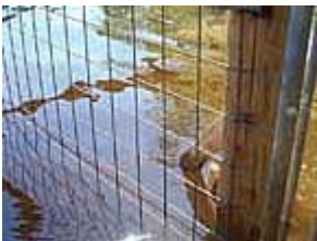
Fence is attached to the corner posts and the bottom of the stringers with staples.
