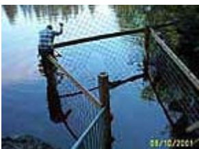
Last section being lowered into place. Note the hole cut out for the pipe to extend through.
