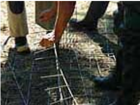
Cutting and bending the fencing material to create a footing.
