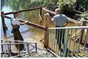
Attaching the stringers to the side posts.
