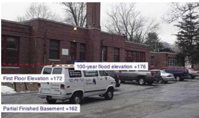
Yorklyn CCArts on a dry day, during floodproofing project. Dotted line shows base flood elevation (BFE), also known as 100-year-flood level.
