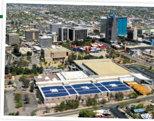
ABOVE: Tucson, Arizona's convention center includes a 591 kilowatt rooftop solar system. Photo courtesy of SPG Solar, Novato, California.
