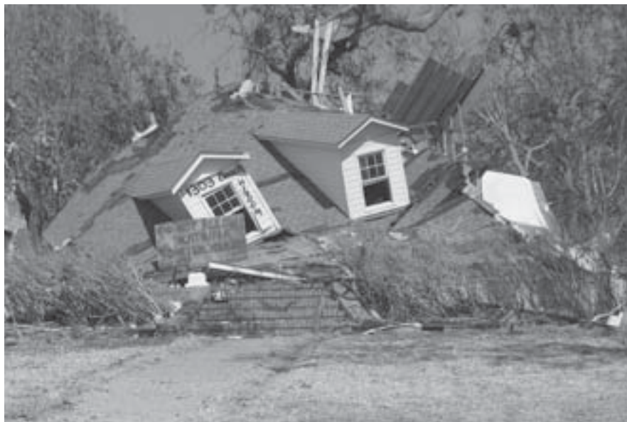
Pascagoula, Mississippi, issued more than 7,500 building permits after Hurricane Katrina to repair and rebuild damaged homes and other structures.
