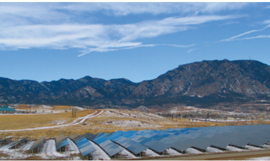
LEFT: At Fort Carson, a 2 MW solar PV facility is sited on a 15-acre decommissioned landfill.
