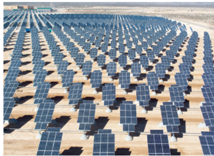
RIGHT: At Nellis Air Force Base, a 14 MW solar PV facility covers 140 acres, including the 33-acre capped landfill.
