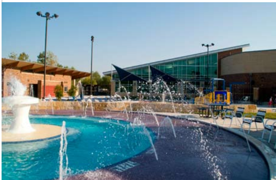
The need for diverse aquatic programs in Plano, Texas, became one of the desired priorities driving the development of its Tom Muehlenbeck Center. The flowing nature and free form of the leisure pool space experience is maximized by a strong visual connection between the inside and outside bodies of water as well as views to the adjacent wetland creek, the shaping force of the project.
