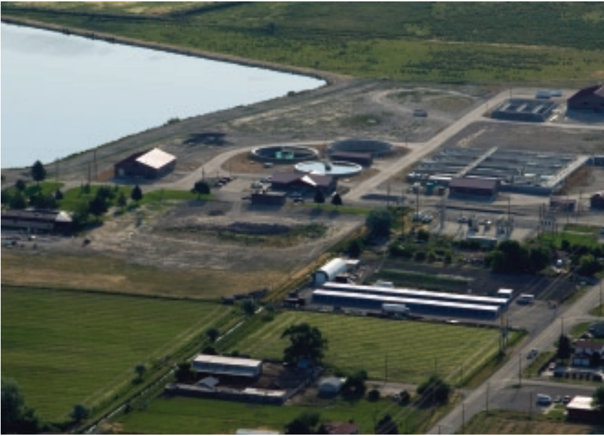
Burley, Idaho's new wastewater treatment facility has stimulated the local economy while providing flexibility to meet strict state and federal regulations.
