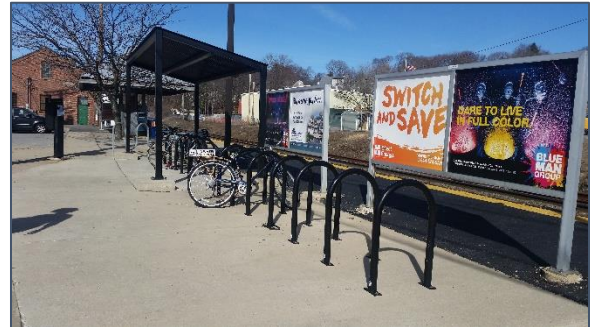
Andover, MA - Transit Station
