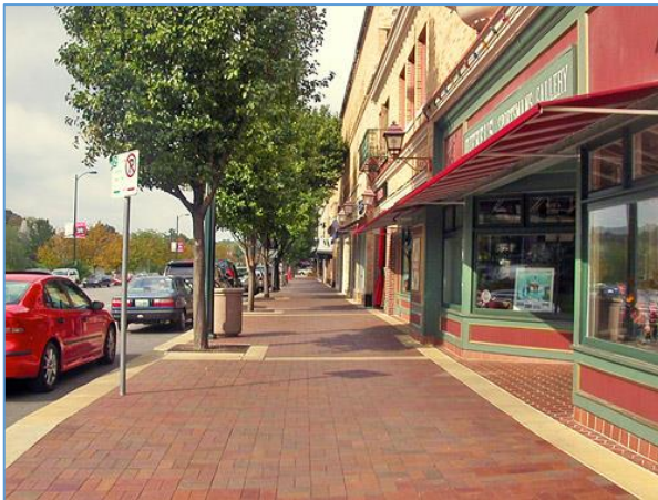
San Francisco, CA - Clean Team Maintains Sidewalks
