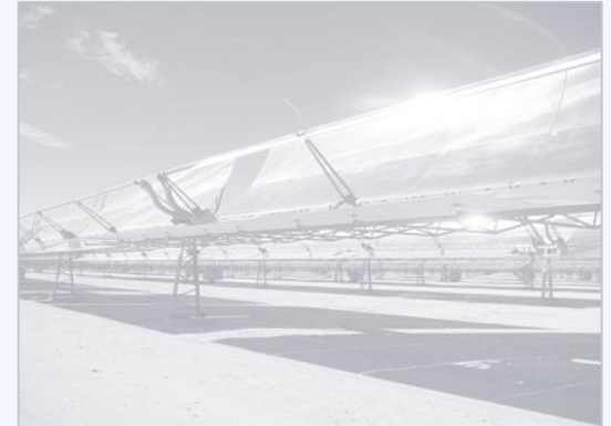
Concentrated Solar Power
