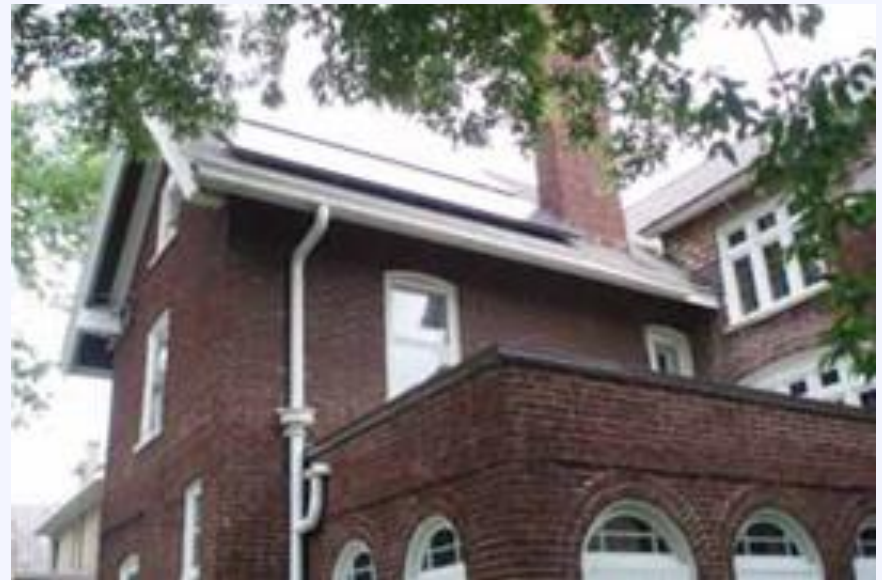
Solar installation on rear of building out of sight from public right of way Heritage Hill Historic District of Grand Rapids, Michigan (Source: Kimberly Kooles, NC Solar Center)
