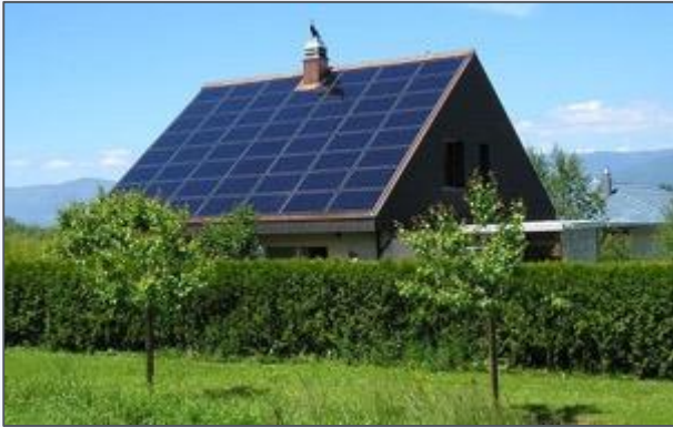
Solar Photovoltaic (PV)
