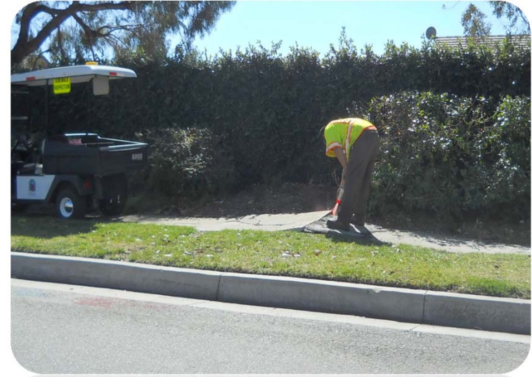
Marking severe hazards with orange highlighted paint
