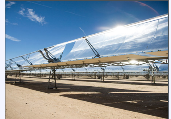
Concentrated Solar Power
