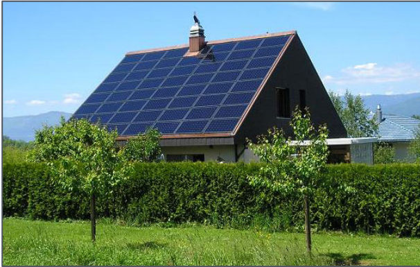
Solar Photovoltaic (PV)
