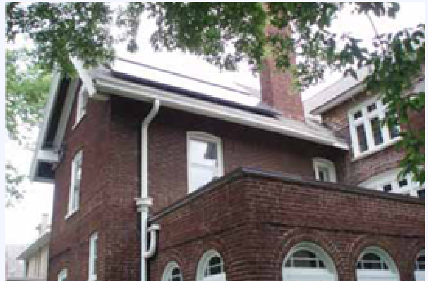
Solar installation on rear of building out of sight from public right of way Heritage Hill Historic District of Grand Rapids, Michigan (Source: Kimberly Kooles, NC Solar Center)
