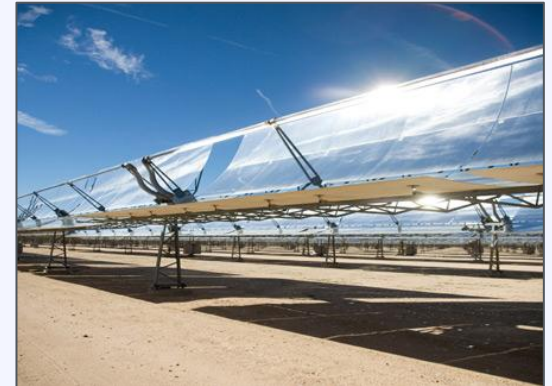
Concentrated Solar Power
