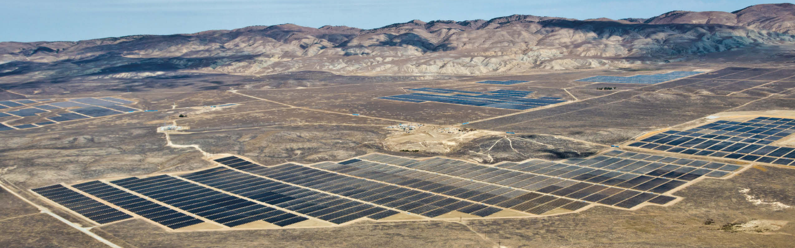
Portion of 250 MW AC California Solar Valley Solar Ranch
