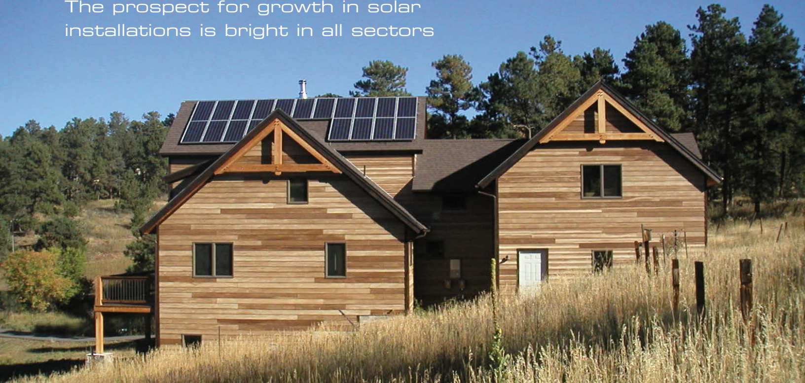
Residential PV Installation in Colorado
