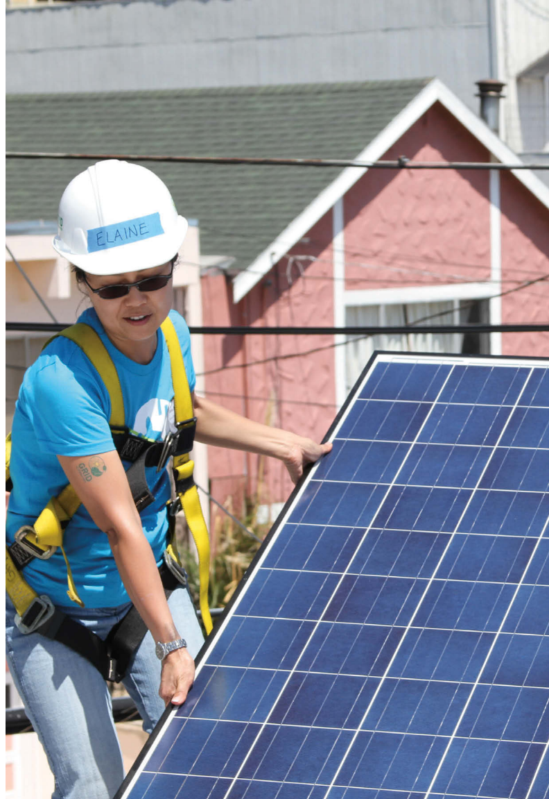
Worker installing PV system
