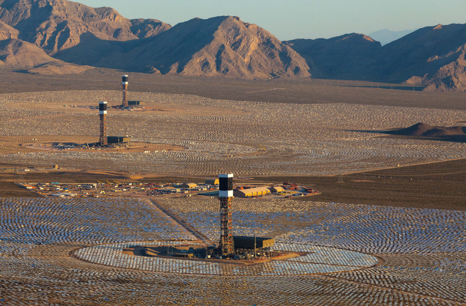
Solar power towers at Ivanpah Solar Electric Generation Station in California
