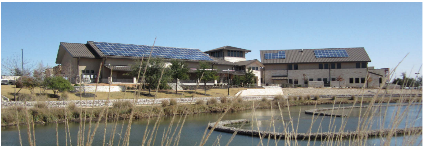
Non-profit PV installation in Austin, Texas
