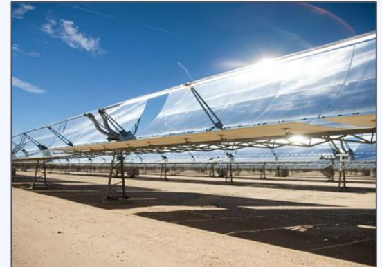
Concentrated Solar Power
