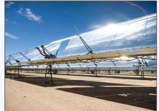
Concentrated Solar Power
