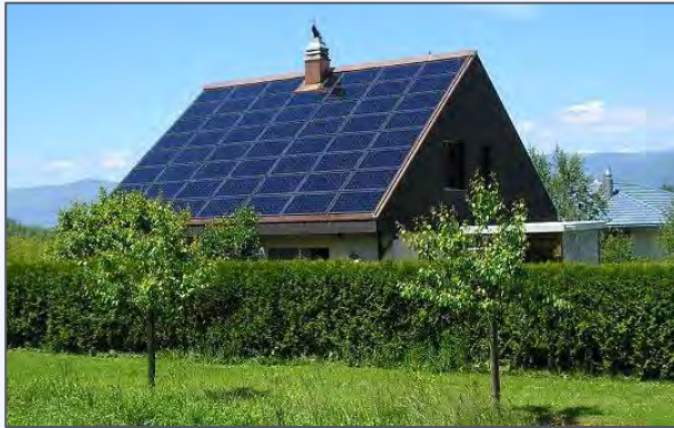
Solar Photovoltaic (PV)
