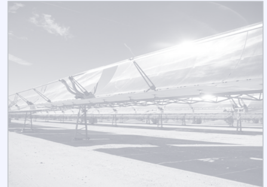
Concentrated Solar Power
