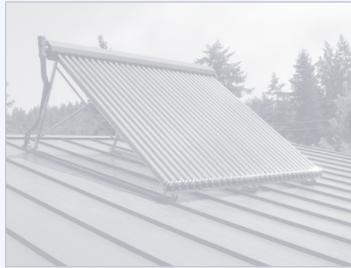
Solar Hot Water
