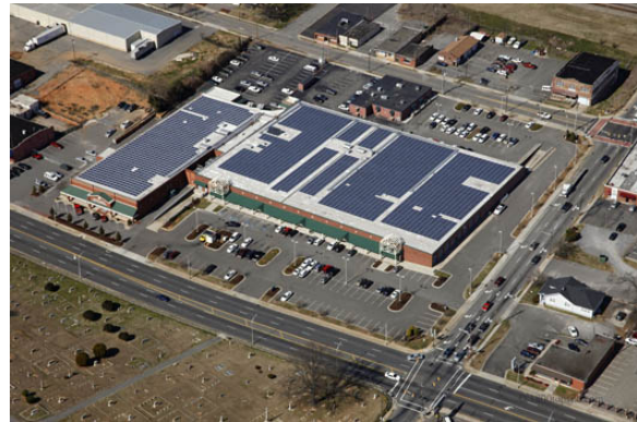
Figure 2- Completed rooftop solar installation on York Chester Plaza building. Photo courtesy of NARENCO.
