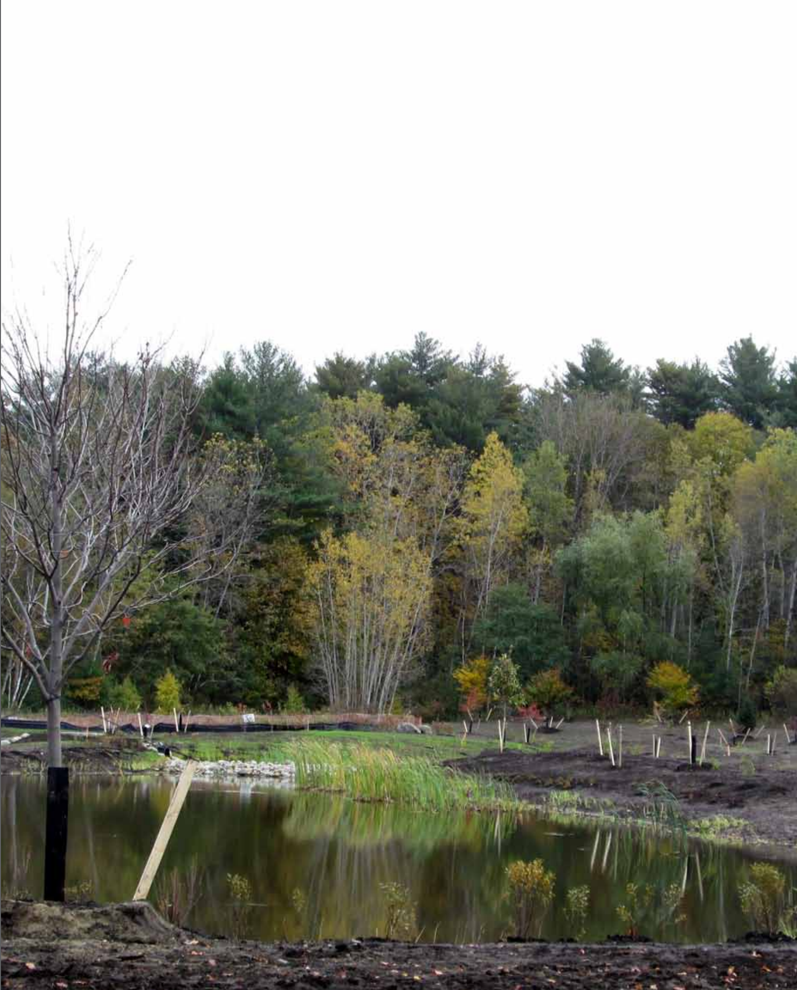
Village of Lake George, West Brook Stormwater Improvement Project
