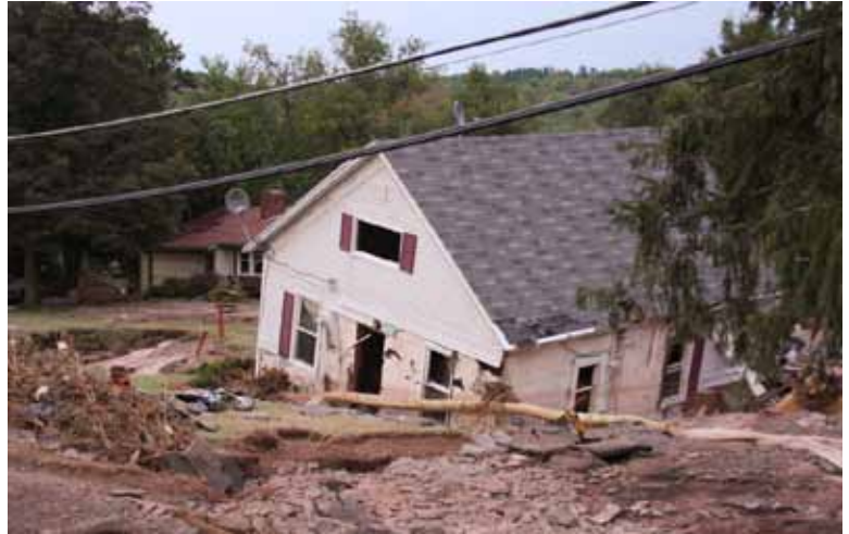
Hurricane Irene damage Town of Prattsville Source: FEMA
