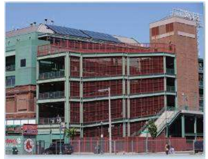
Solar water heating system installed by goSolar on Fenway Park provides one third of the stadium's hot water. Courtesy: Boston Red Sox
