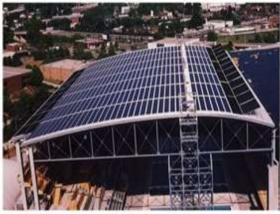
Solar water heating system installed by goSolar on Fenway Park provides one third of the stadium's hot water. Courtesy: Boston Red Sox
