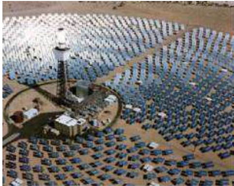
Central Receiver or Power Tower
