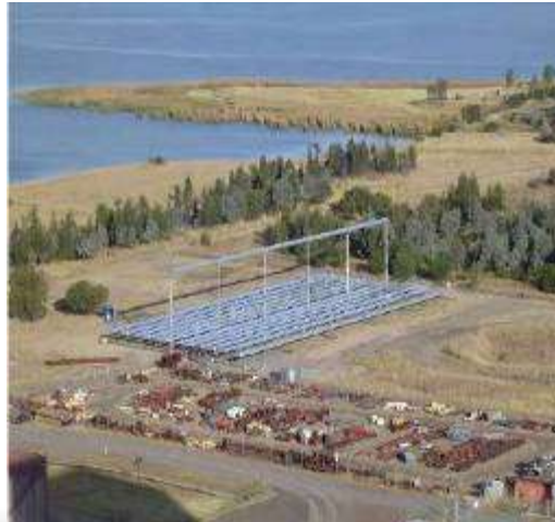
Compact linear Fresnel reflector
