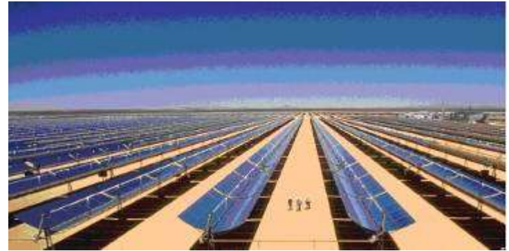
Parabolic trough
