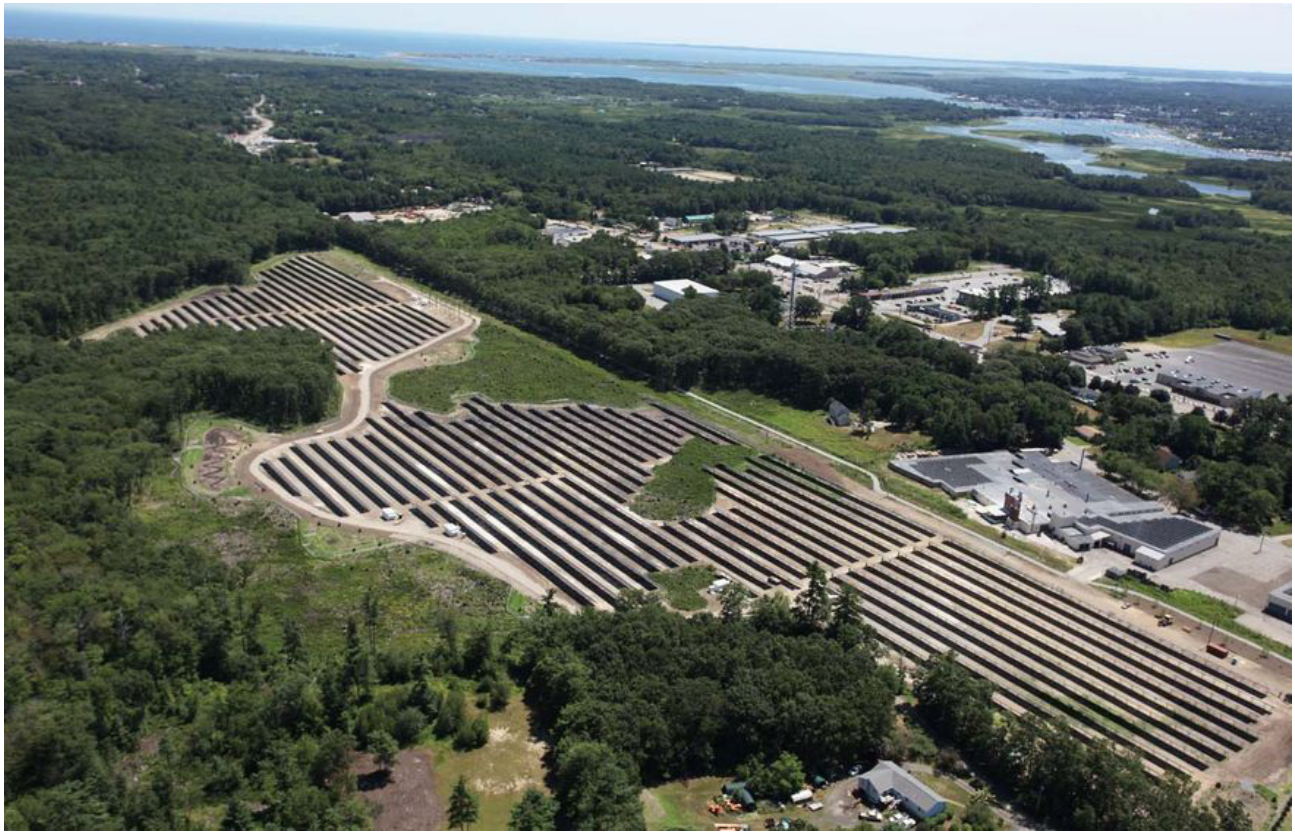
Photo Credit: Salisbury Solar Farm
