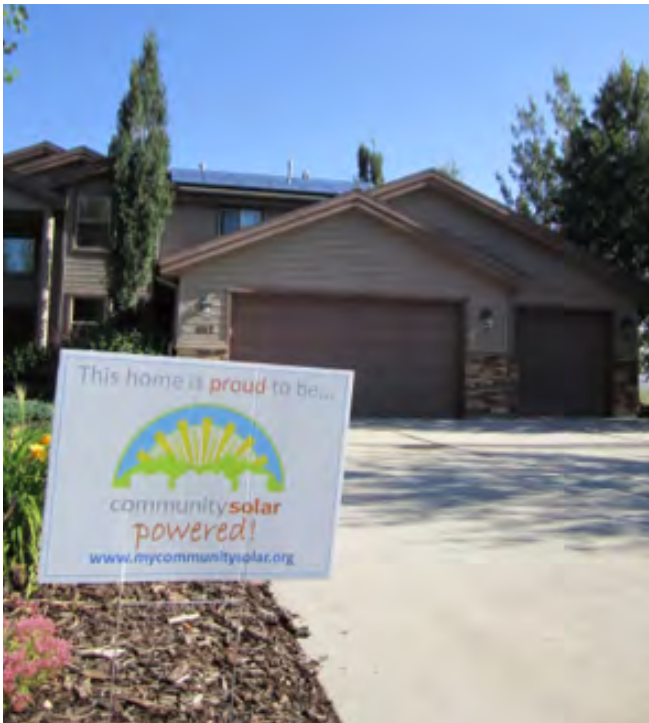
Solar photovoltaic panels installed as part of the Summit Community Solar program. Photo credit: Alpenglow Solar.
