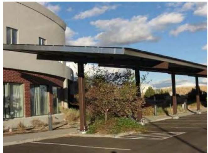
Solar shade parking structure at fire station #11, Reno, NV 5
