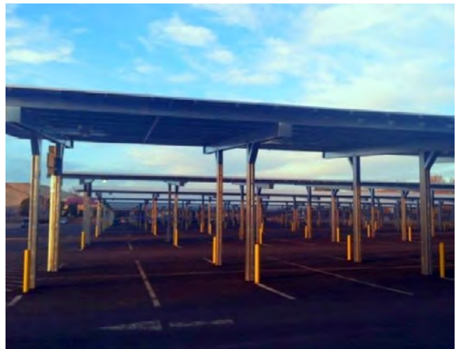
Solar parking shade structure at Reed High School, Reno NV 8
