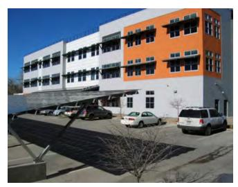
The Innosphere project includes a 44-kilowatt photovoltaic (PV) system installed on the carport. The owner of this office building used the commercial PV rebate to help fund the project in 2011. Photo Credit: City of Fort Collins
