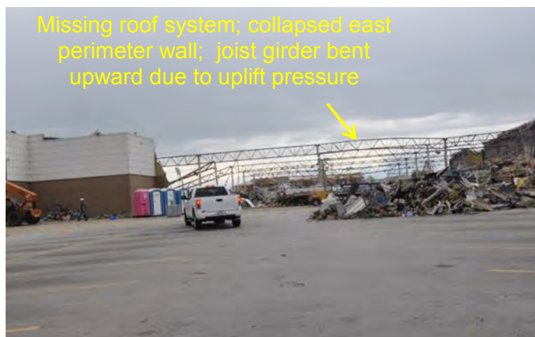
Figure 3–38. Large area of roof system shown missing. Joist girders bent upward due to uplift pressure.
