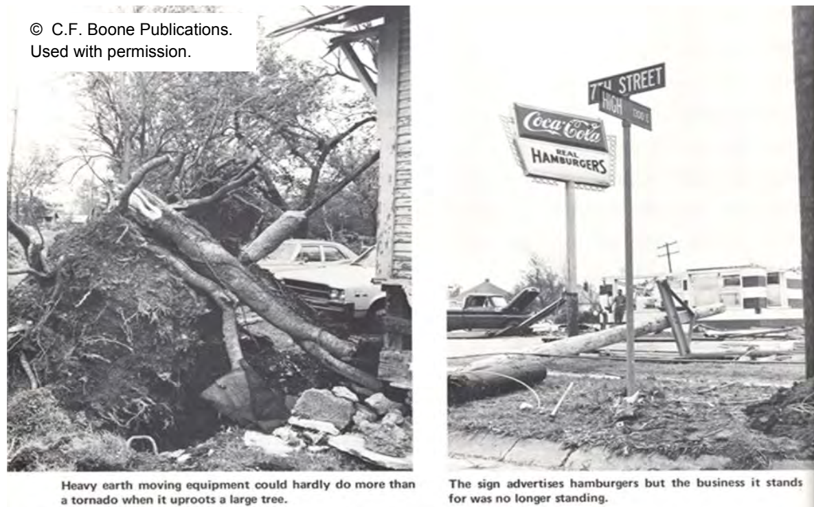
Figure 1–3. Damage from the 1971 Joplin tornado. 31
