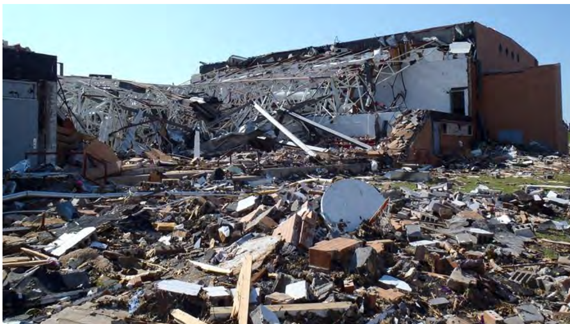
Figure 3–69. View from west of the Joplin High School Gymnasium building.
