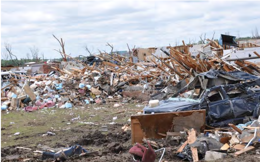
Figure 3–105. Collapsed Greenbriar Nursing Home.
