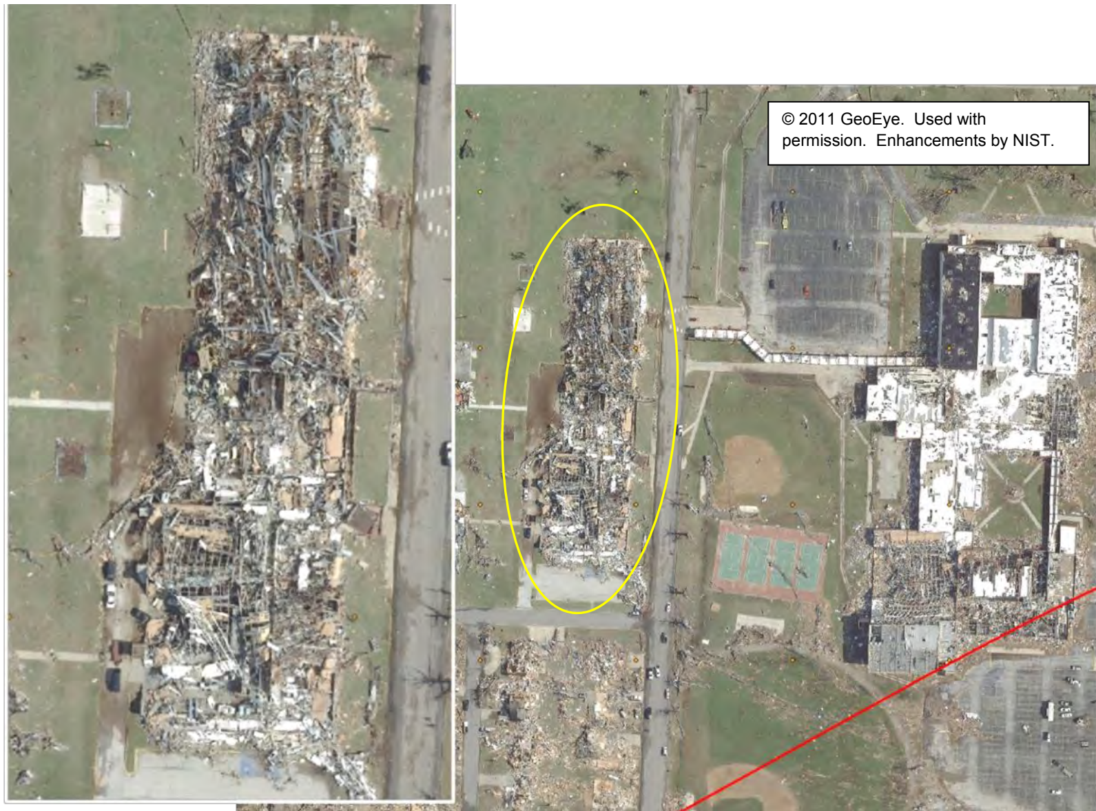
Figure 3–74. Overview of damage at Franklin Technology Center, with center line of tornado damage path (in red).
