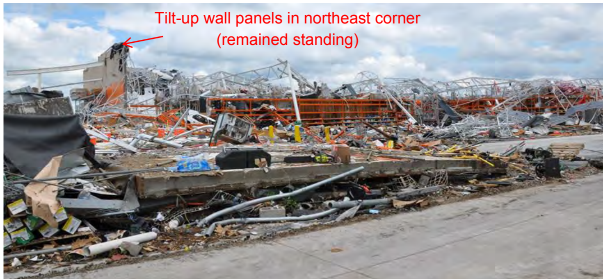
Figure 3–49. Collapsed Home Depot building (view from the northwest). Note the loss of all roof decks and upward displacement of joists and joist-girders
