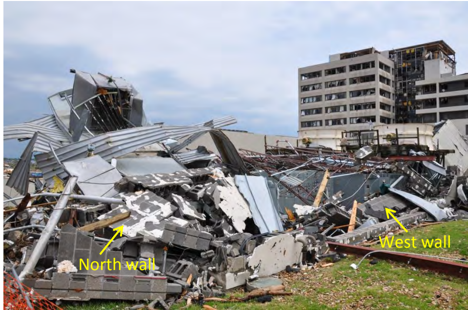
Figure 3–20. View from northwest of Emergency Generator Building. Note northward and eastward direction of wall failure, consistent with the direction of maximum wind (westerly) shown on Figure 3–7.
