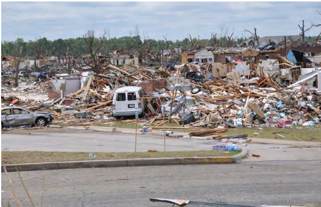
Figure 3–104. Collapsed Greenbriar Nursing Home (viewed from the east) with missing roof system and collapsed exterior CMU walls. Note debris from building materials as well as other sources (automobiles) in all interior areas of the facility.
