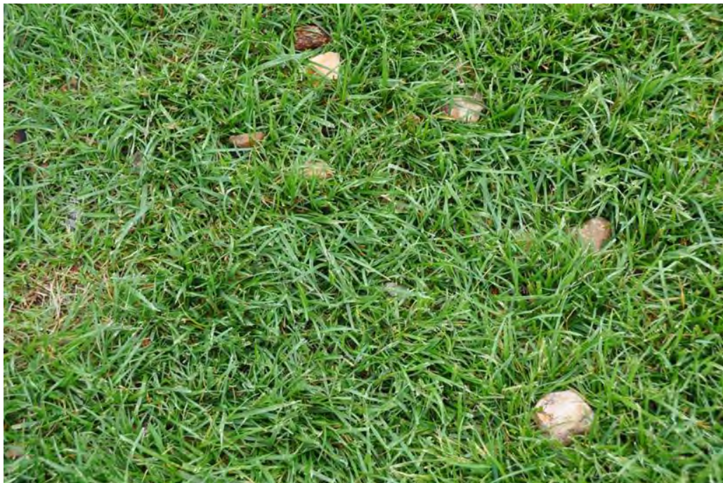
Figure 3–31. Roof aggregate ballast became wind-borne debris (on ground by Medical Office Building 2).
