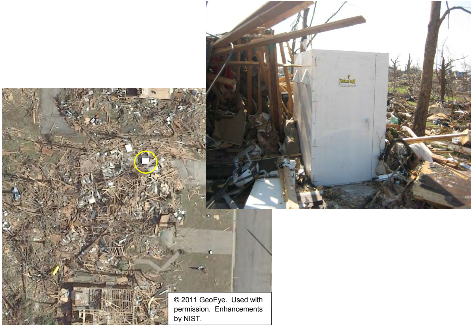
Figure 3–128. Wood–frame home completely destroyed except for the steel shelter bolted to the concrete floor in the garage.
