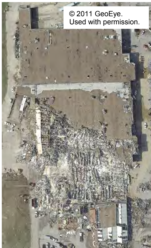
Figure 2–13. Aerial photo of Walmart Store #59 showing extensive damage to the southern (bottom) half of the building.
