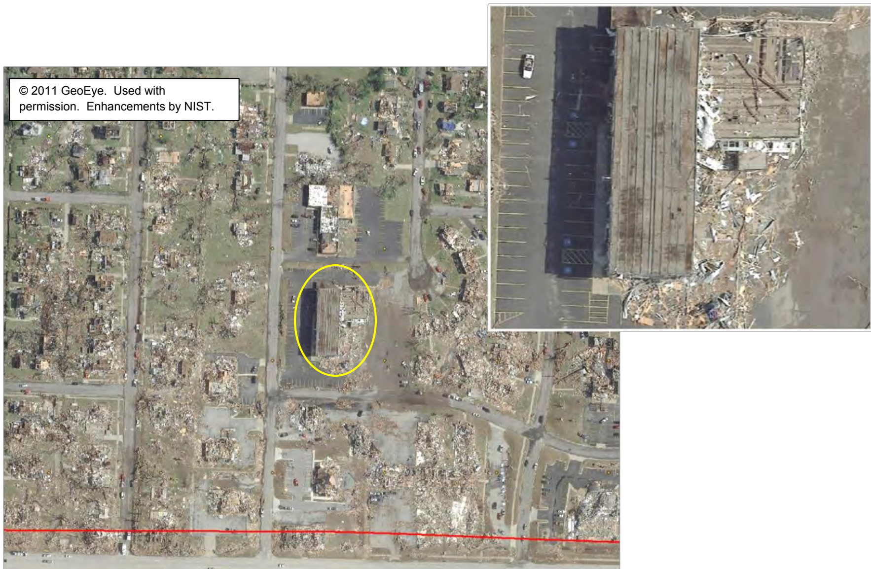
Figure 3–84. Overview of damage to the Ozark Center for Autism and surrounding buildings, with estimated center line of tornado damage path shown in red.
