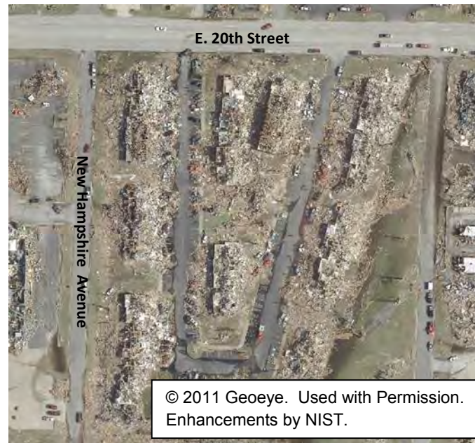
Figure 4–38. Aerial photo showing damage to the Hampshire Terrace apartments.
