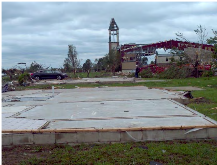
Figure 4-14. Demolished home located within the tornado damage path in Joplin.
