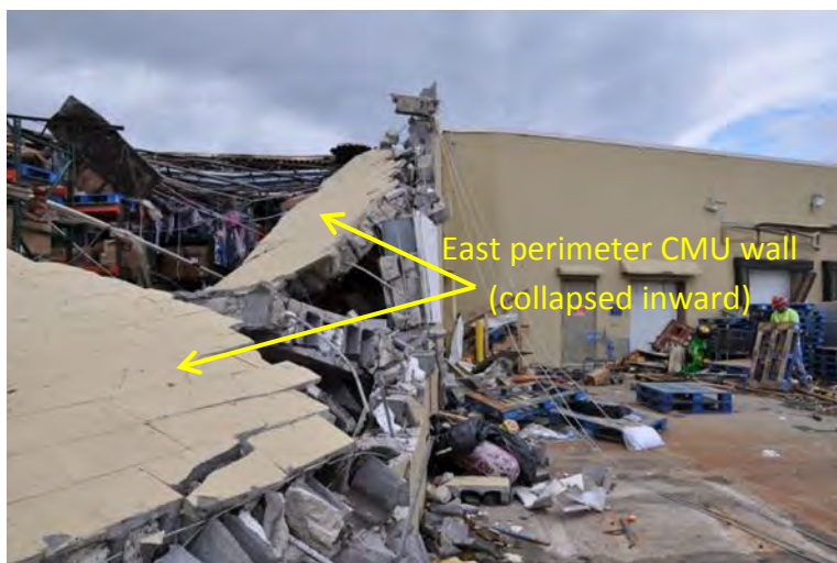
Figure 3–40. Collapsed east wall due to loss of roof lateral bracing and inward wind pressure.
