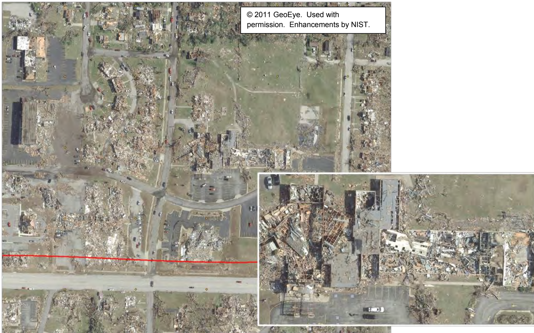
Figure 3–80. Overview of damage at St. Mary’s Catholic Elementary School, with estimated center line of tornado damage path shown in red.
