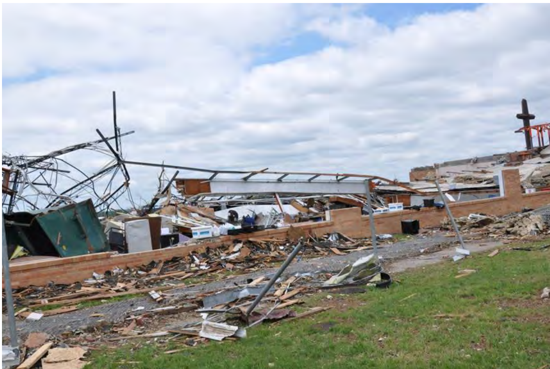
Figure 3–83. Section of building at St. Mary’s Catholic Elementary school with collapsed perimeter CMU walls.
