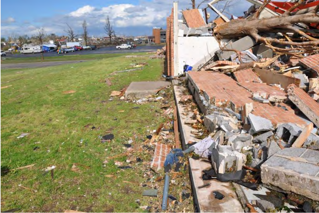
Figure 3–78. Perimeter CMU wall that collapsed after loss of roof lateral bracing (note lack of reinforcing dowels connecting wall to concrete footing).
