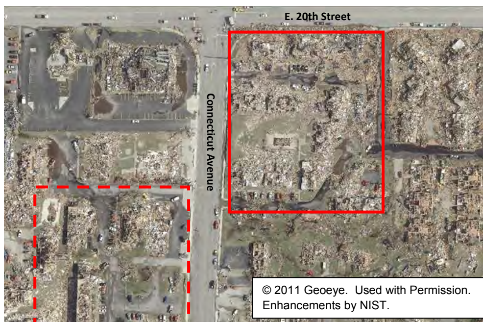
Figure 4–37. Aerial photo showing damage to two apartment complexes in Joplin at 2001 Connecticut Avenue (outlined by solid red line) and 2034 Connecticut Avenue (within dotted line).
