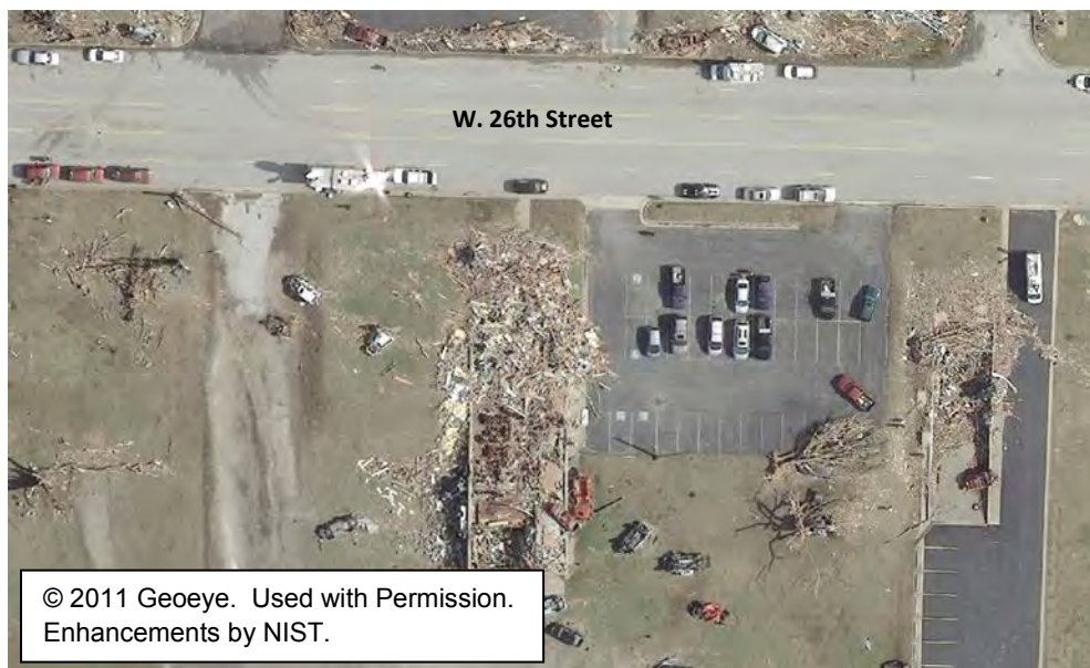
Figure 4–32. Aerial photo showing damage to the Stained Glass Theater.
