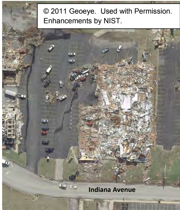
Figure 4–30. Aerial photo showing damage to Harmony Heights Baptist Church.
