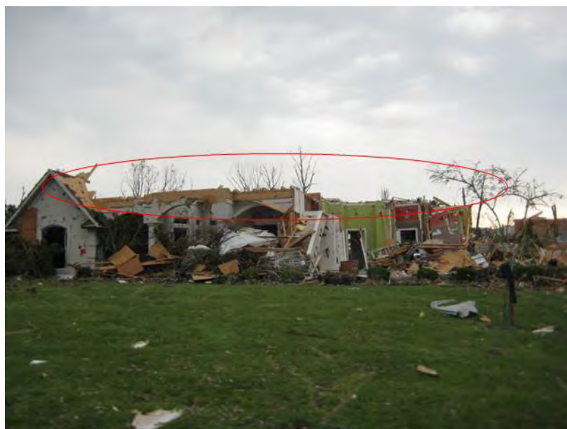
Figure 3–116. Typical roof-to-wall connection damage.
