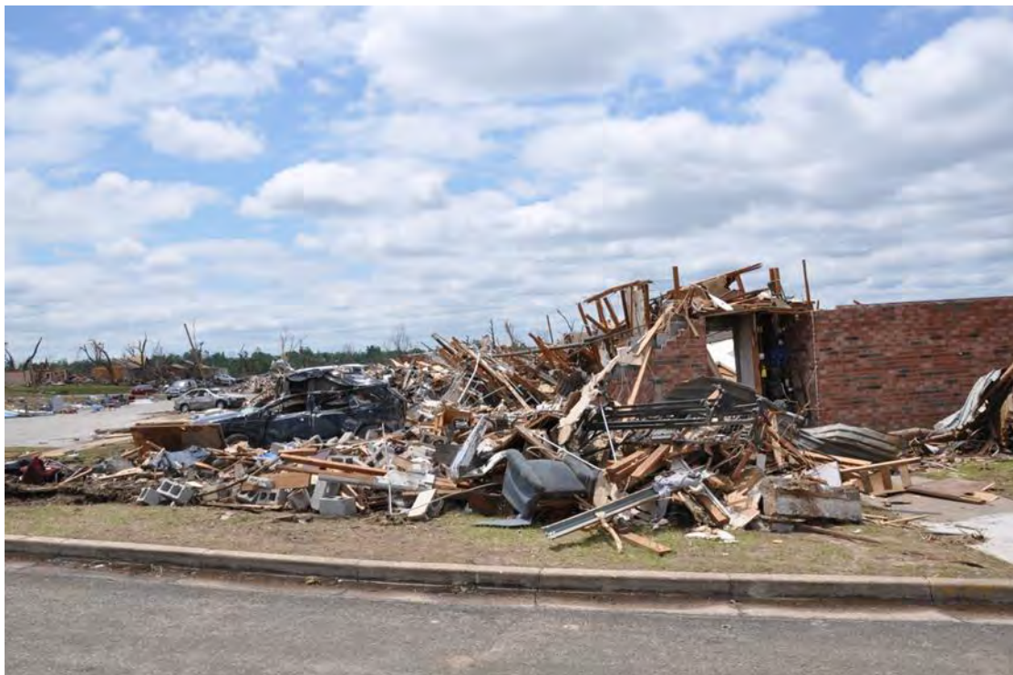
Figure 3–106. Collapsed Greenbriar Nursing Home (viewed from the north) showing the portion of the north wing’s exterior wall that did not collapse.
