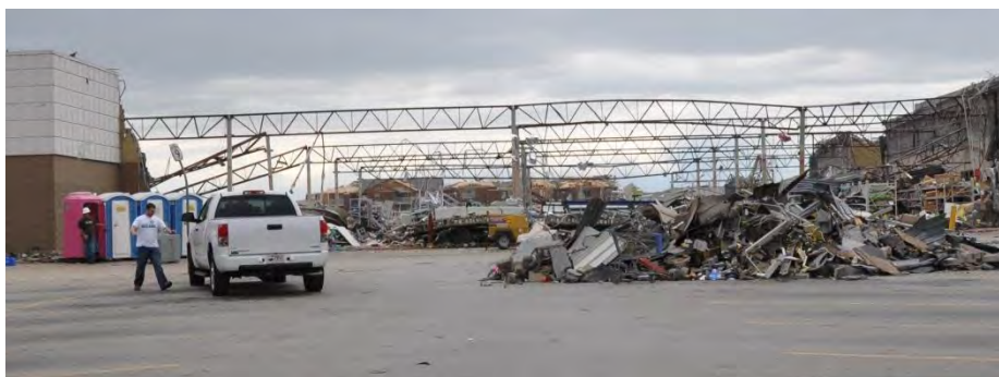
Figure 2–14. Elevation view of southwest-facing wall of Walmart Store #59.
