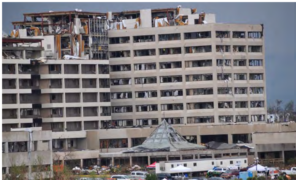
Figure 3–14. View from southwest of East Tower showing that most windows on south and west sides of building and curtain walls on connecting elevator steel frame have broken.
