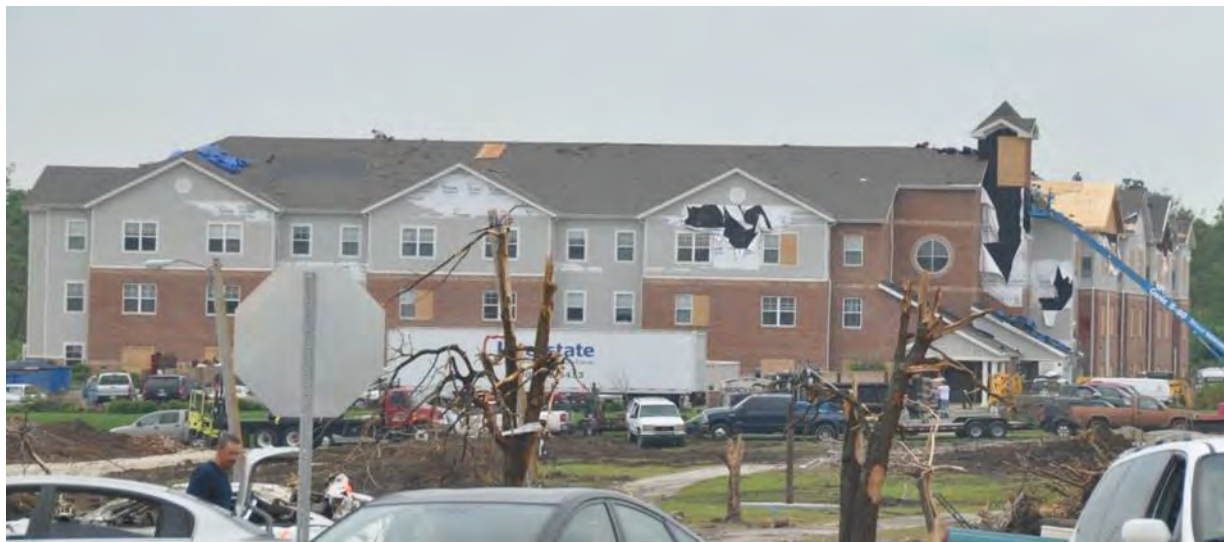
Figure 3–111. Mercy Village Apartments, viewed from the north, with envelope damage (sidings, window glazing, roof covering).
