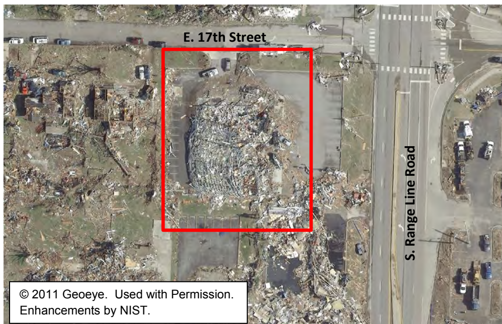
Figure 4–27. Aerial photo showing the AT&T store demolished by the storm (outlined in red).
