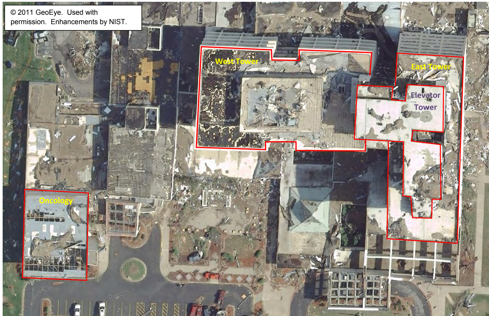
Figure 3–19. Overview of West, East, and Elevator Towers and Oncology Clinic Building showing that most of the aggregates that were used as roof ballast on these buildings are missing.
