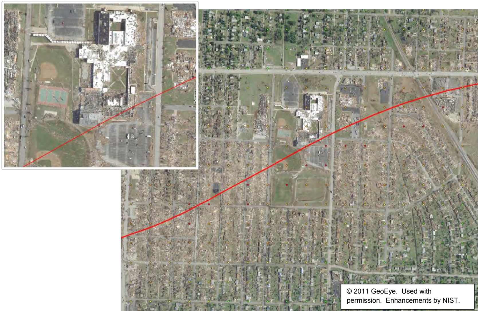
Figure 3–64. Overview of Joplin High School complex, with estimated center line of Joplin tornado damage path shown in red.
