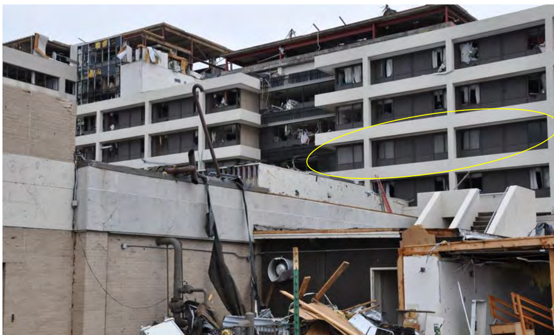
Figure 3–11. Intact windows on fifth floor of West Tower (north side).
