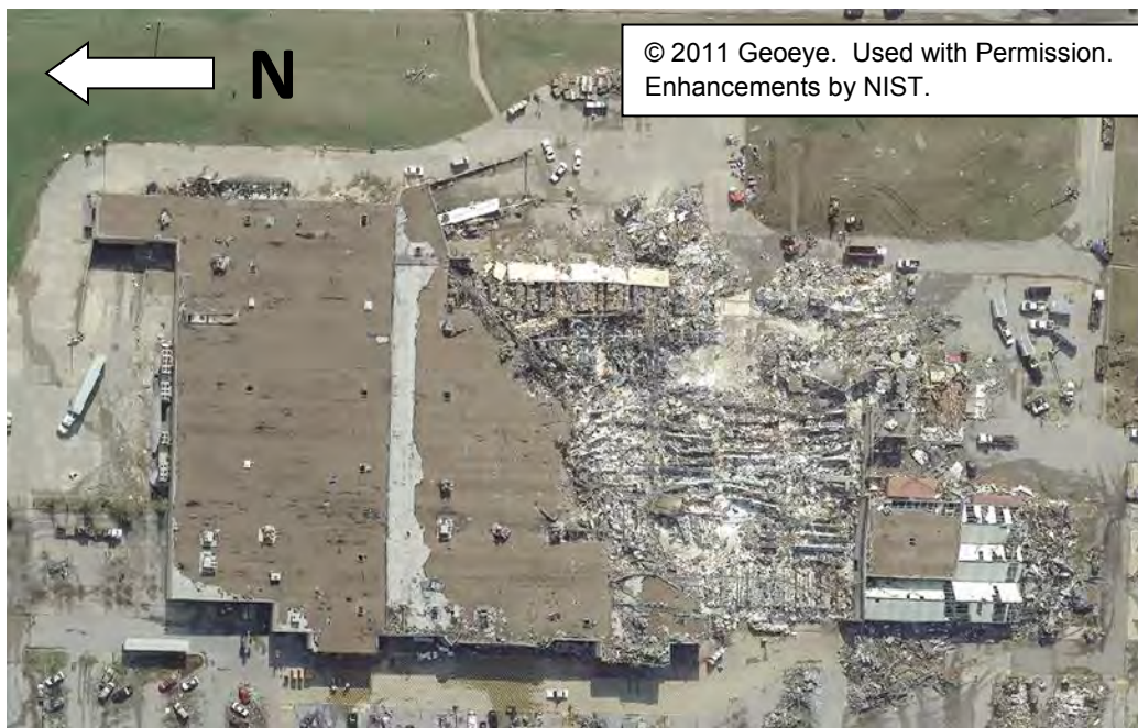
Figure 4-12. Aerial photo of the tornado-damaged Walmart Store #59, showing the collapsed south half and uncollapsed north half of the building.
