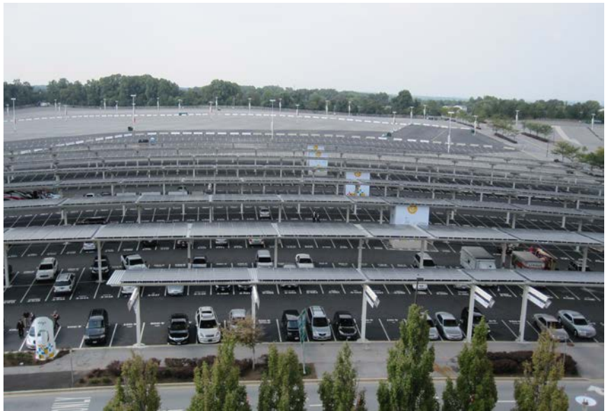
Solar Panels at FedEx Field.
