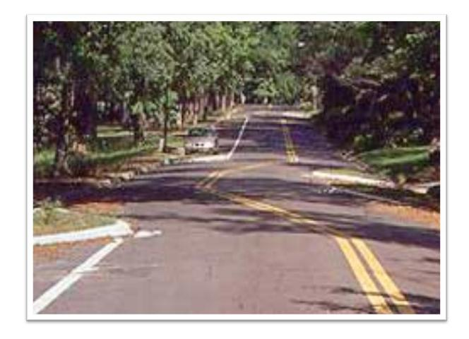
Chicanes are a type of horizontal deflection used to reduce the speed of traffic as drivers are expected to reduce speed to negotiate the lateral displacement in the vehicle path.
