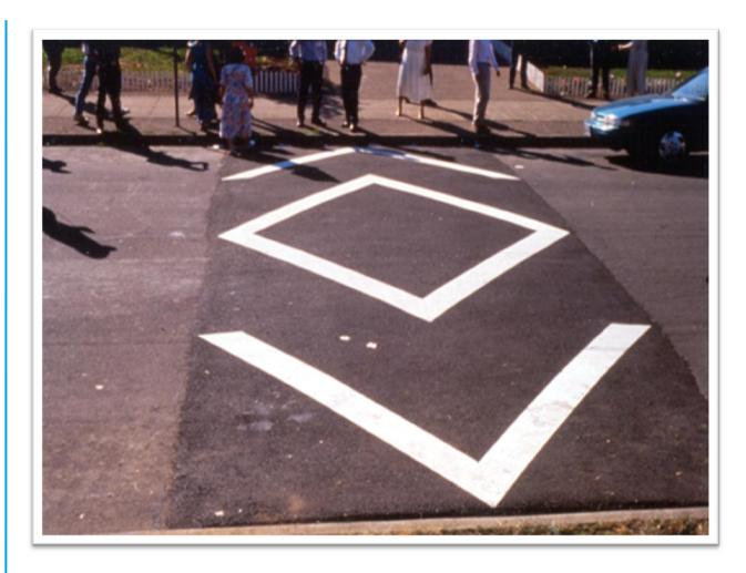
Speed humps are rounded, raised areas placed across the street which are usually visually marked and designed to slow traffic as vehicles travel over the hump.
