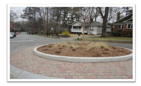
Traffic calming measures, such as mini-circles, medians, bulb-outs, and speed humps reduce vehicular speeds by:
