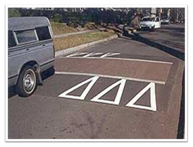
Speed tables contain flat top, raised surfaces that generally allow a car to be fully on the raised surface before exiting the speed table.
