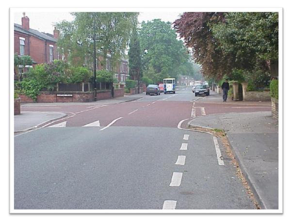
This traffic calming measure raises an entire intersection with elevated approaches from all directions. The raised intersection may include sidewalk crossings near the intersection and it is very useful in areas with high pedestrian traffic.
