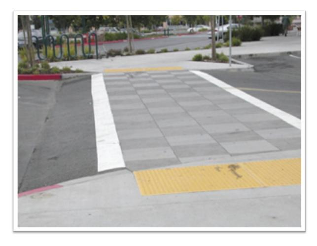
A raised crosswalk is essentially a speed table outfitted with crosswalk markings and signage to channelize pedestrian crossings. Raised crosswalks are useful mid-block away from intersections.
