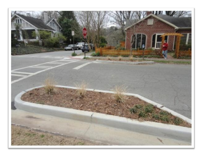
Bulb-outs narrow driver sight distance as they physically narrow roadway width.
