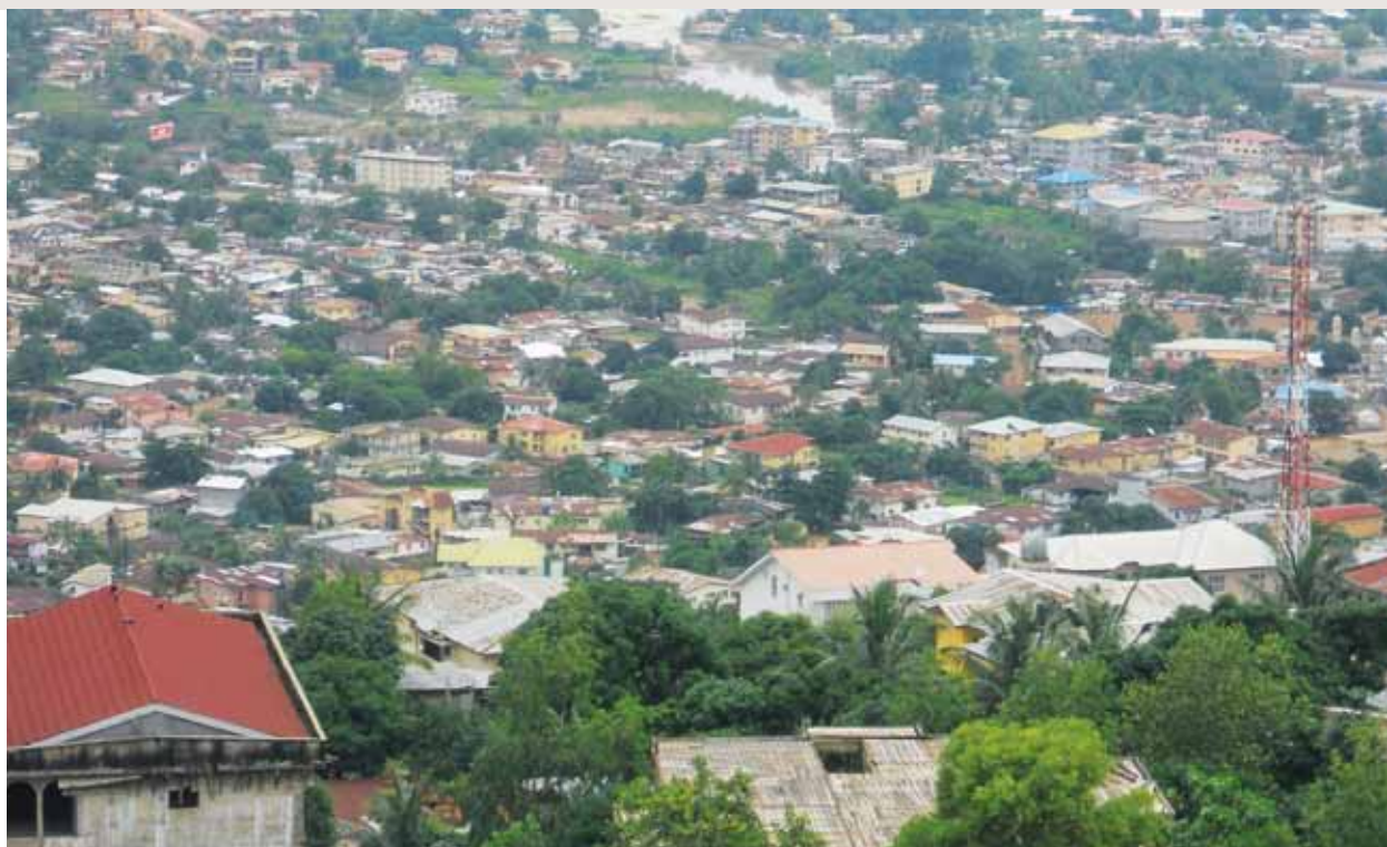
Constructions in low-lying areas in Freetown damaged by flooding Photo: Marielle Dubbeling
