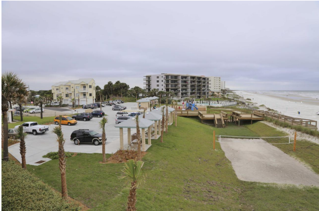
ESTHER STREET BEACHFRONT PARK AFTER CONSTRUCTION
