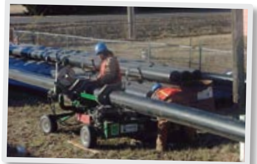
Constructing the Maize Public Water System.
