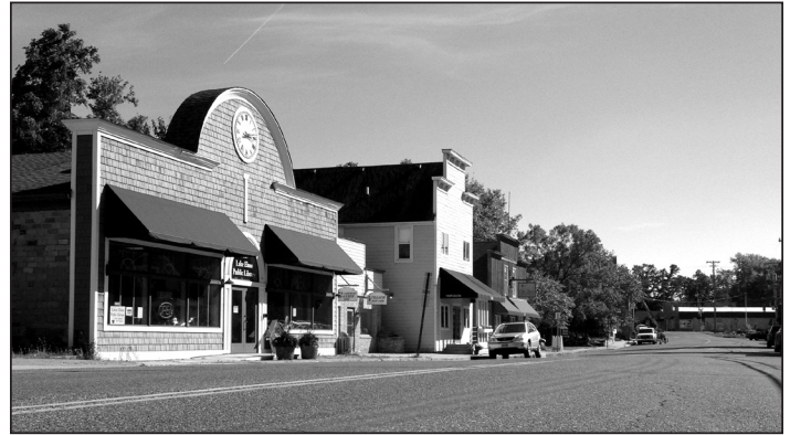
Construction for improvements to downtown Lake Elmo is targeted for construction in 2015.
