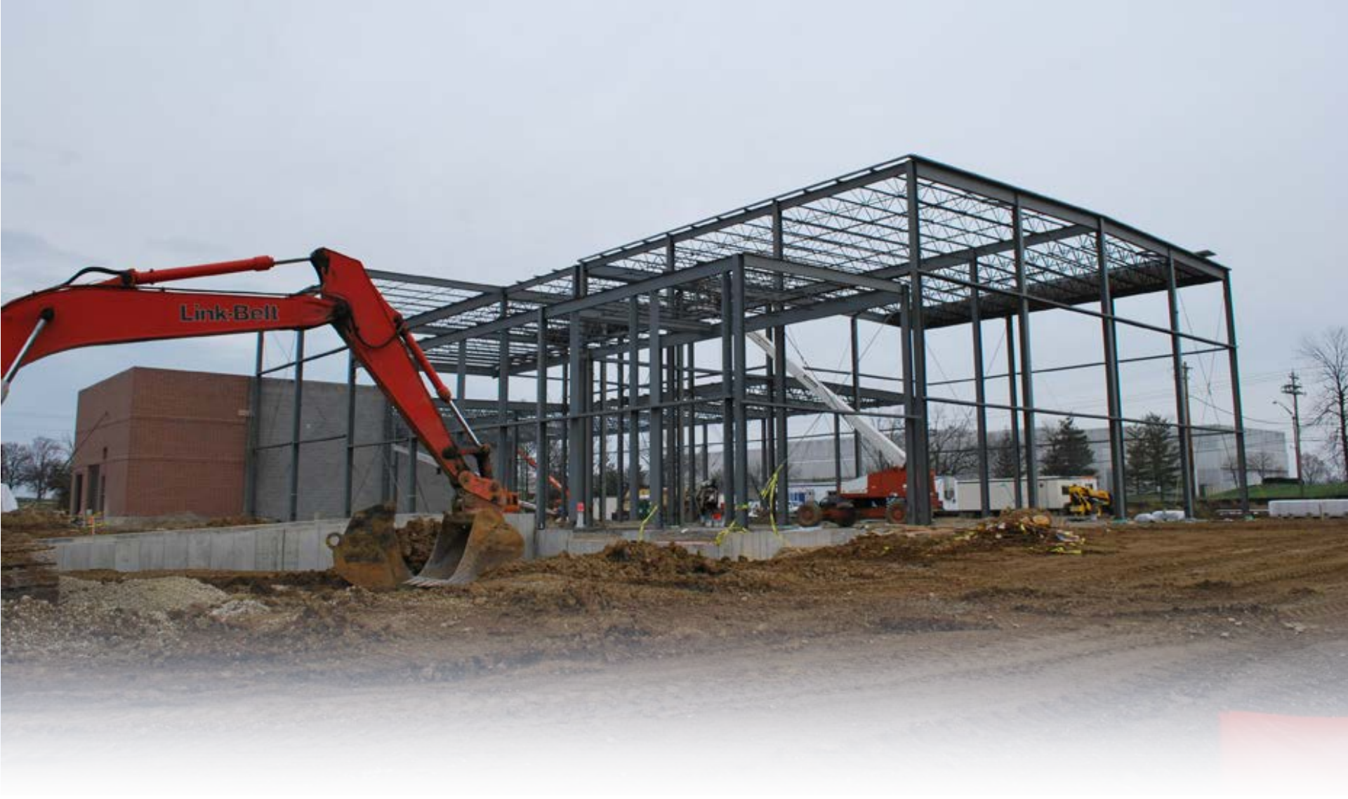
Graeter's facility (under construction)
