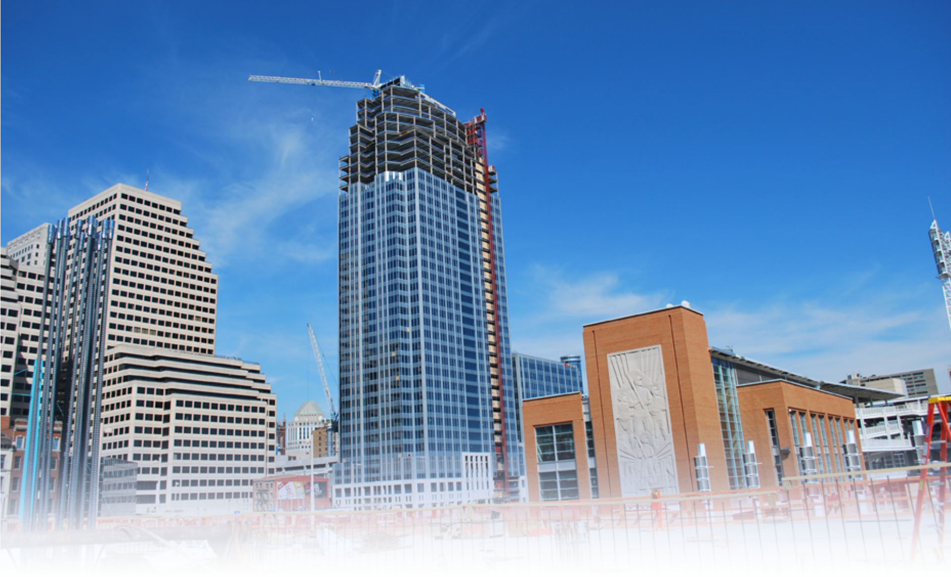
Great American Tower (under construction)
