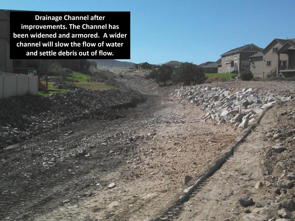
Culverts (that were plugged with debris) were removed opening up the channel to the detention basin and preventing future spillover onto residential properties.
