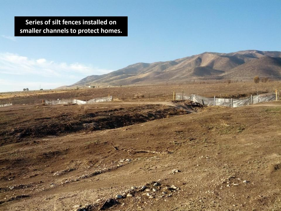
Silt fence. Includes one field fence and one chain link fence with a heavy duty fabric liner. These fences will hold water back and prevent debris flow.
