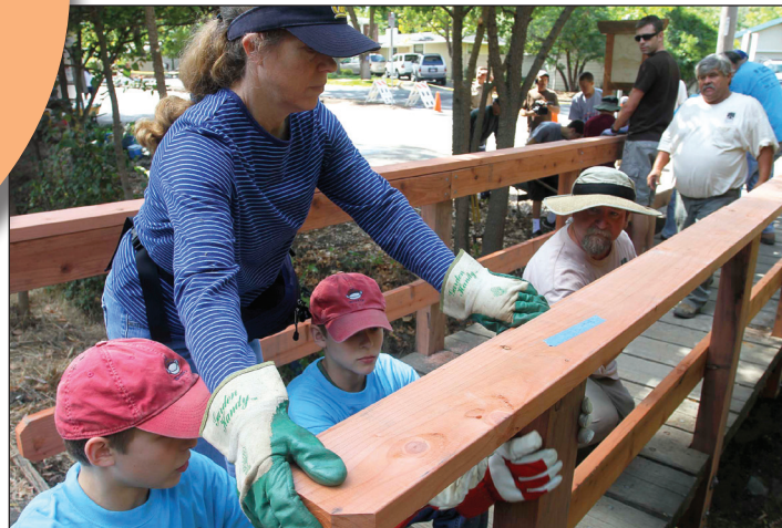
Volunteers of all ages teamed up to make Walnut Creek a better place at the first Community Service Day on October 1, 2011. Here, volunteers build a bridge at the Howe Homestead park. The 2012 Community Service Day will be Saturday, Oct. 6.
