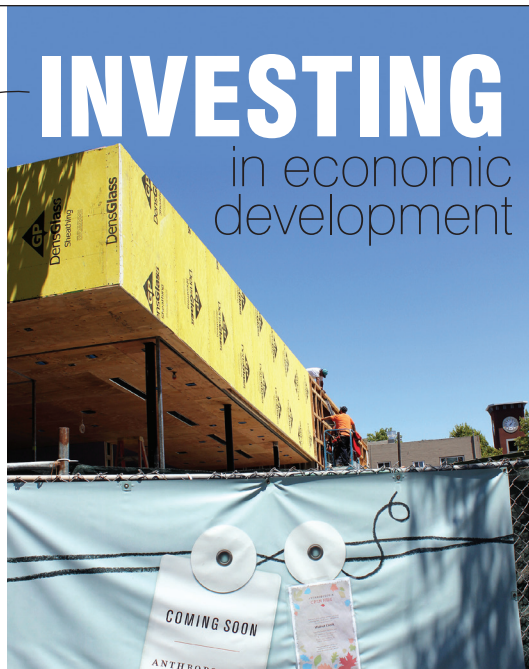
Construction of Anthropologie is under way in downtown.
