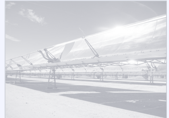
Concentrated Solar Power
