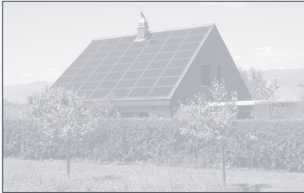
Solar Photovoltaic (PV)
