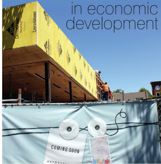
Construction of Anthropologie is under way in downtown.
