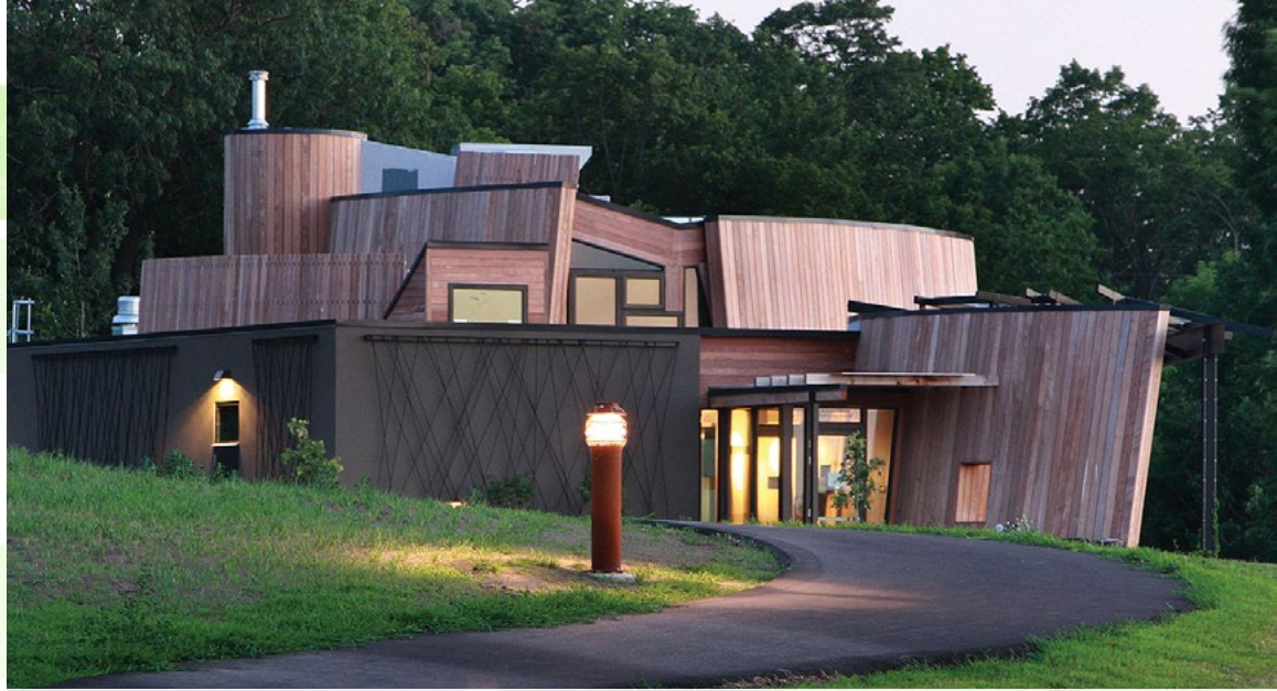
The Gathering Center at Spring Lake Park generates nearly all of its annual electricity needs – often sending excess power back to the grid – using a nearby wind turbine. Indoor temperature is controlled through super insulation techniques and automated shading devices. The building captures rainwater to flush toilets, and then treats the water on-site. Photo courtesy of Dakota County.
