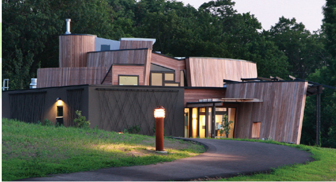
The Gathering Center at Spring Lake Park generates nearly all of its annual electricity needs – often sending excess power back to the grid – using a nearby wind turbine. Indoor temperature is controlled through super insulation techniques and automated shading devices. The building captures rainwater to flush toilets, and then treats the water on-site. Photo courtesy of Dakota County.
