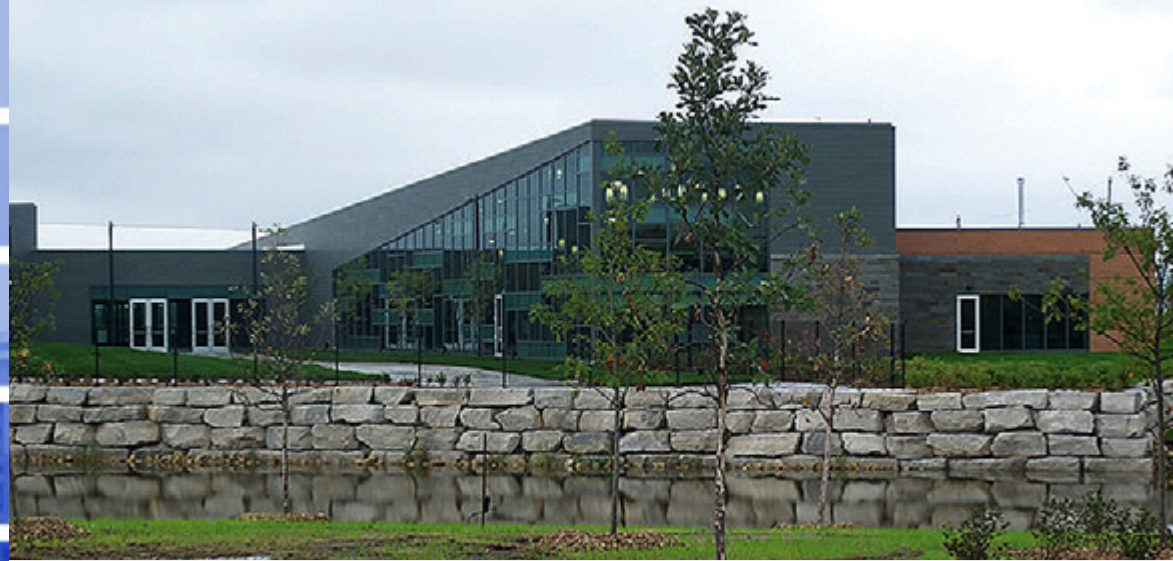
This remodeled Washington County, Minn. library has been designed to be as energy efficient and sustainable as possible through the use of natural ventilation, day lighting, selection of materials, energy efficient lighting and mechanical units, and controls to monitor and adjust for use and time.
