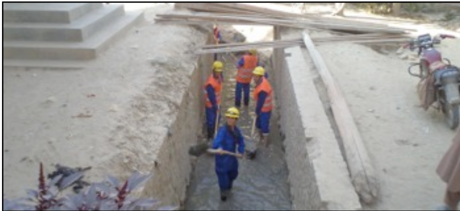
Locally-hired day laborers work to clean mud and other debris from Sar-e-Pul canals.
