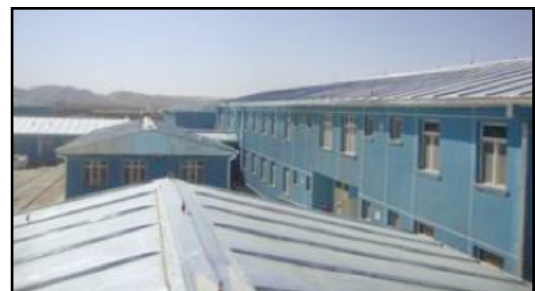
The newly built Provincial Teacher Training College in Faryab.
