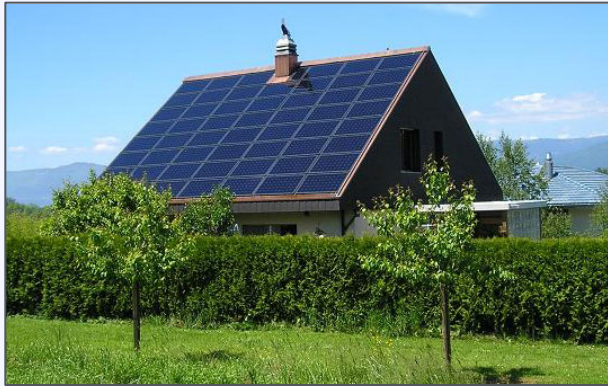
Solar Photovoltaic (PV)
