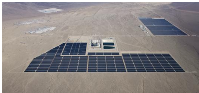
Copper Mountain Solar Project near Boulder City, Nevada Photo courtesy of First Solar
