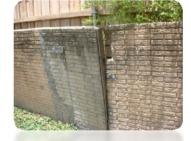
resorted to reinforcing the wall with steel bars in the ground to prevent it from collapsing into his backyard. The City's code enforcement division began issuing code notices to homeowners along the wall because the condition of the wall was so deteriorated that it was no longer code compliant.
