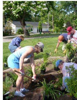
MCLA rain garden digging
