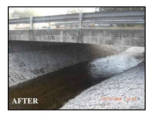
Gee Creek at Gee Creek Lane Project: The existing private concrete retaining wall behind a home was overtopped by the creek flows, eroding and undermining the retaining wall. Additionally, a storm sewer outfall that discharges into the creek collapsed. Funding provided by NRCS was used to build a protective wall of gabion rock and replace the storm sewer that collapsed. The private properties adjacent to the creek are now protected from further erosion.
