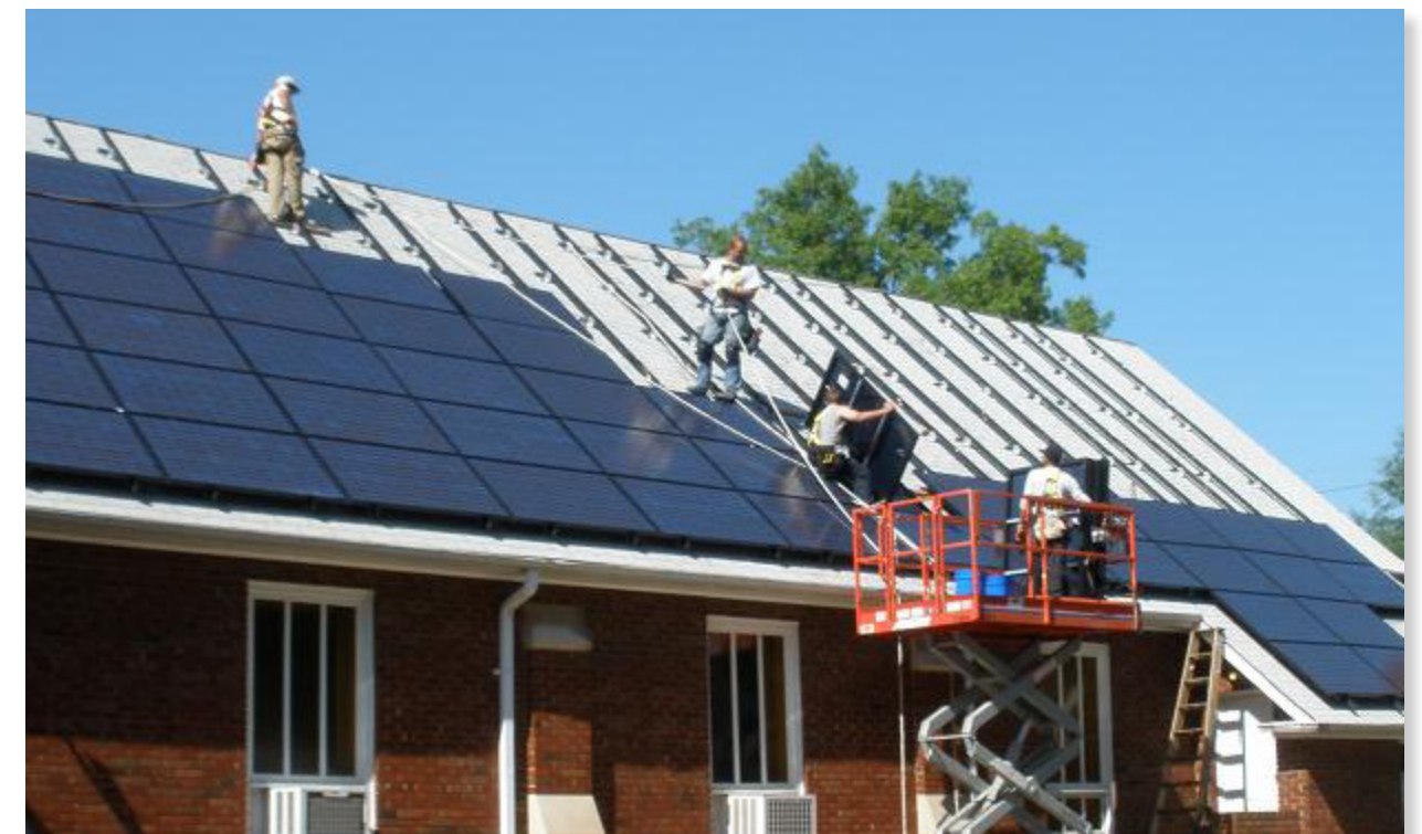
Installing Panels on the Church of the Brethren, University Park, Maryland
